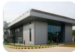
Eco Commercial Building (ECB) Bayer Material Science, Greater Noida, UP
