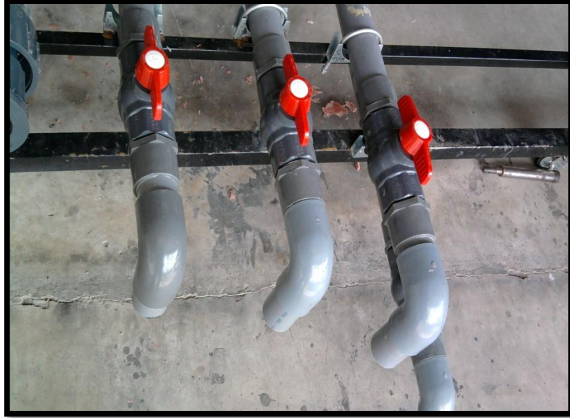
Figure A.24: Drain system
