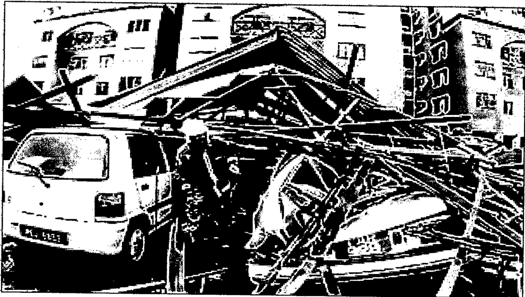
Figure 1.1: Apartment Roof Falling Down on Vehicles (Arkib Utusan, 2004)
