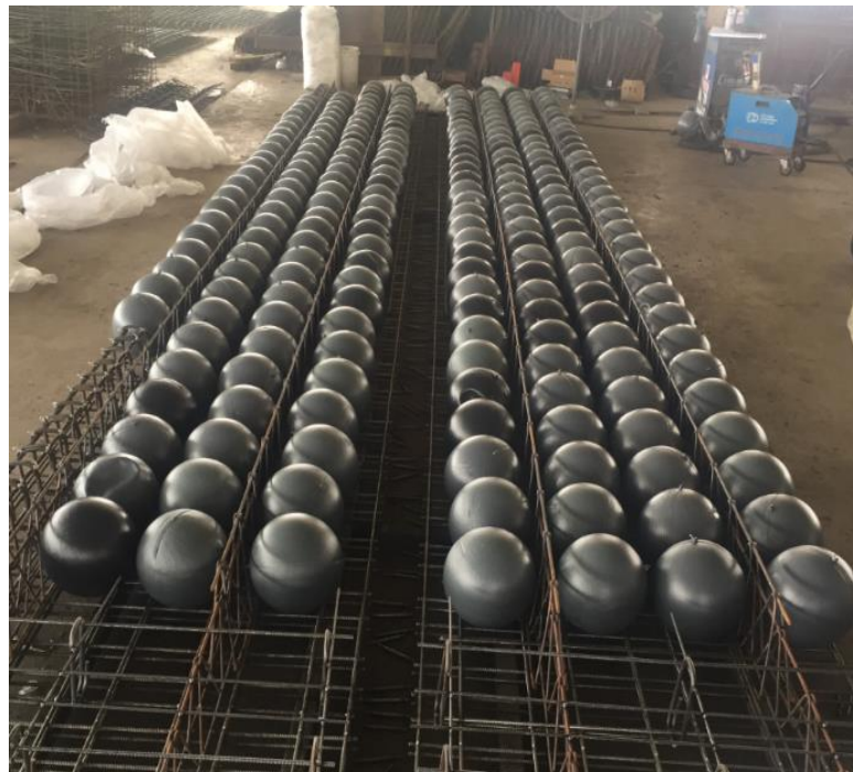
Figure 3.2 HDPE plastic hollow bubbles
