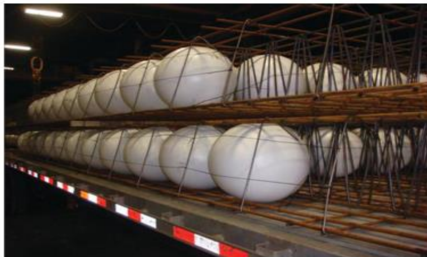
Figure 2.1 Plastic spheres along with reinforcement
