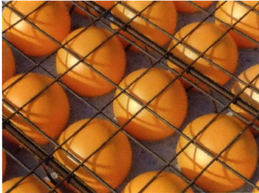
Figure 1.3 Components of a bubble deck slab
