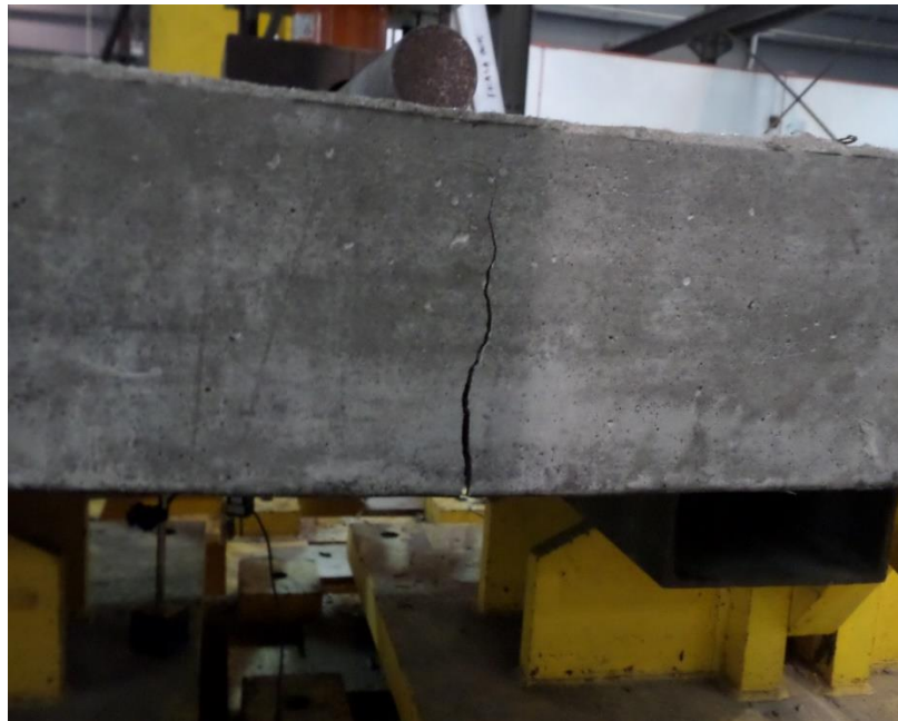
Figure 4.9 Crack initiated at the middle of slab sample
