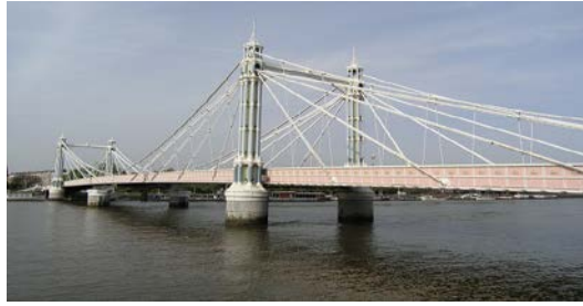
Figure 2.4 Albert Bridge, built in 1872. (Inge Kanakaris-Wirtl, 2009)
