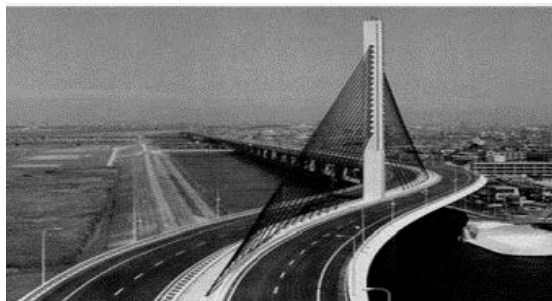
Figure 2.14 S Curve of Katsuhika Harp Bridge (Dionysius M.Siringoringo, 2007)
