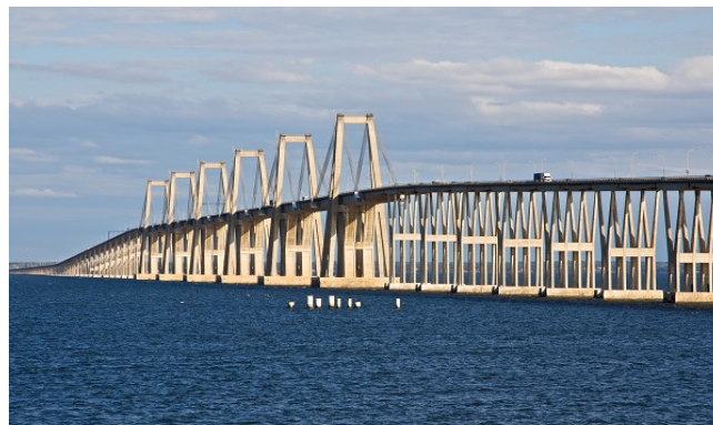
Figure 2.22 General Rafael Urdaneta Bridge in Venezuela (Orlando Pozo, 2009)
