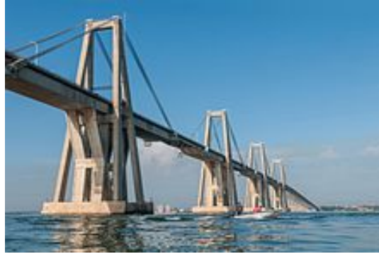
Figure 2.8 General Rafael Urdaneta Bridge at Venezuela
