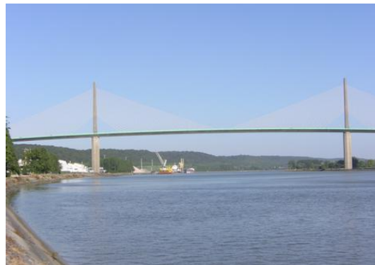
Figure 2.9 Brotonne bridge (Pont de Brotonne) in France
