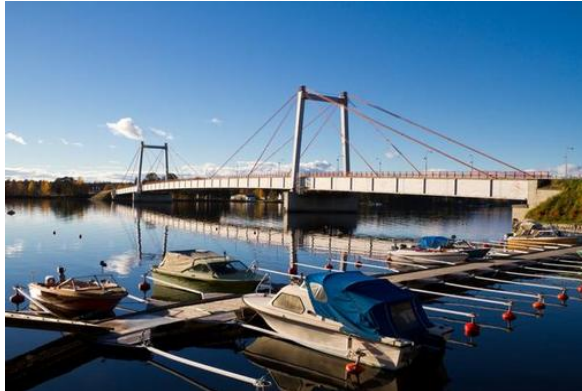
Figure 2.6 Strömsund Bridge at Sweden (Lars Falkdalen, 1955)
