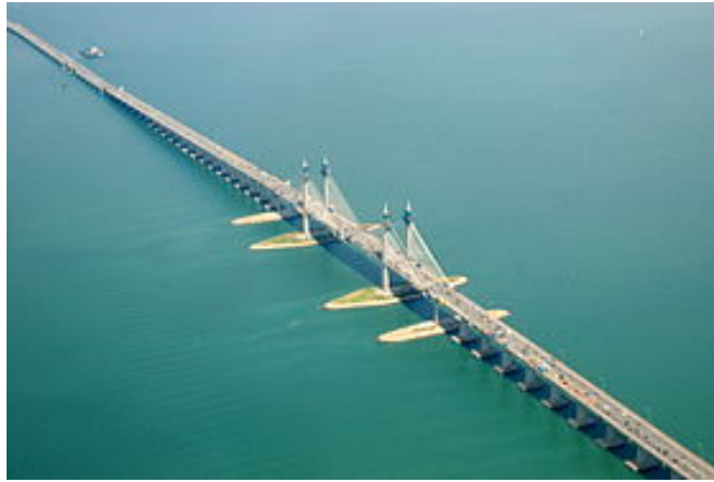
Figure 3.2 The Sultan Abdul Halim Muadzam Shah Bridge
