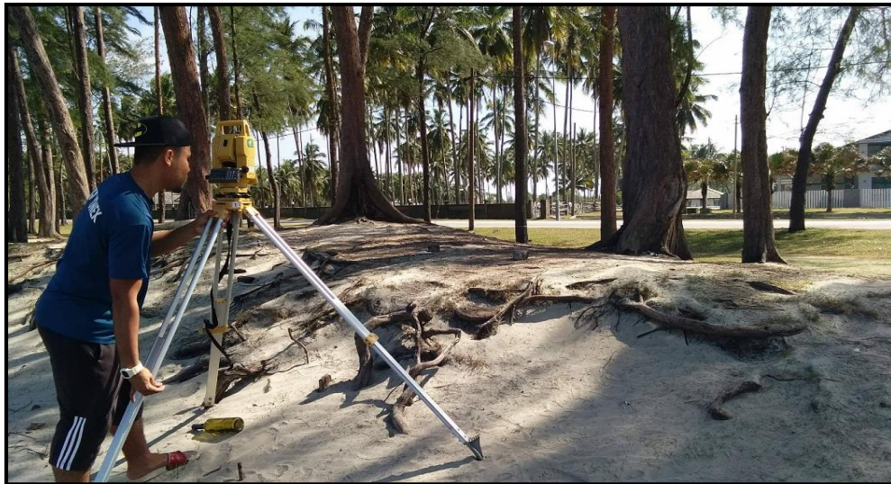
Figure 3.4 Surveying work at Pantai Sepat
