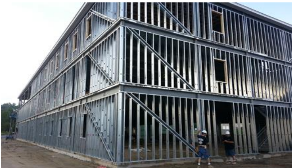
Figure 1.2 Uses of CFS framing
