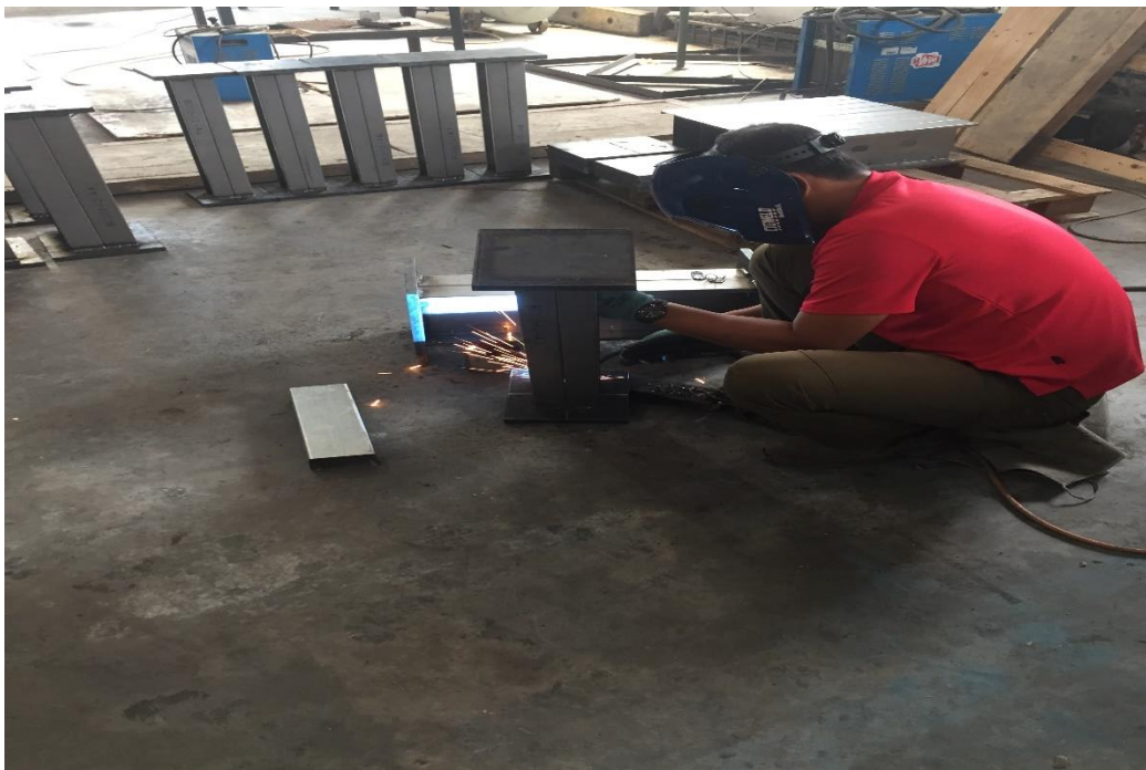
Figure 3.5 Welding the Base Plate to be Fixed-Ends
