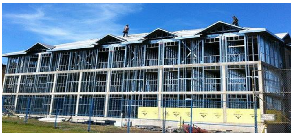
Figure 2.2 Roof system using cold-formed Source: Moen & Schafer (2008).
