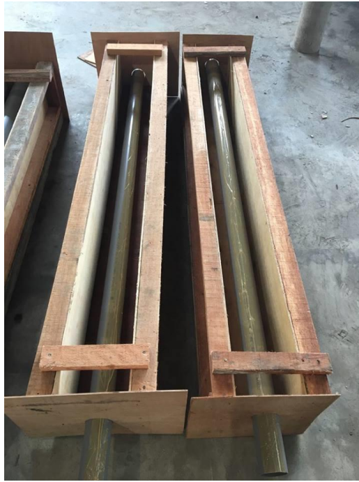
Figure 3.2 Preparation of Formwork
