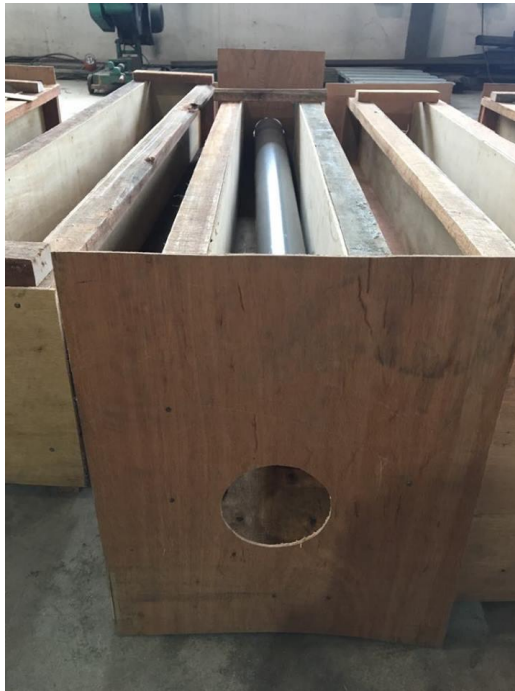
Figure 3.3 Circular Hollow Section Formwork
