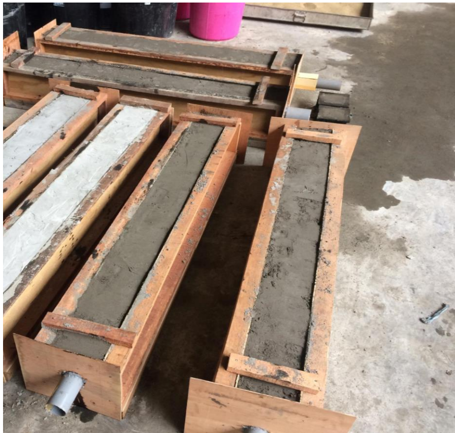
Figure 3.8 Casting of the Specimen
