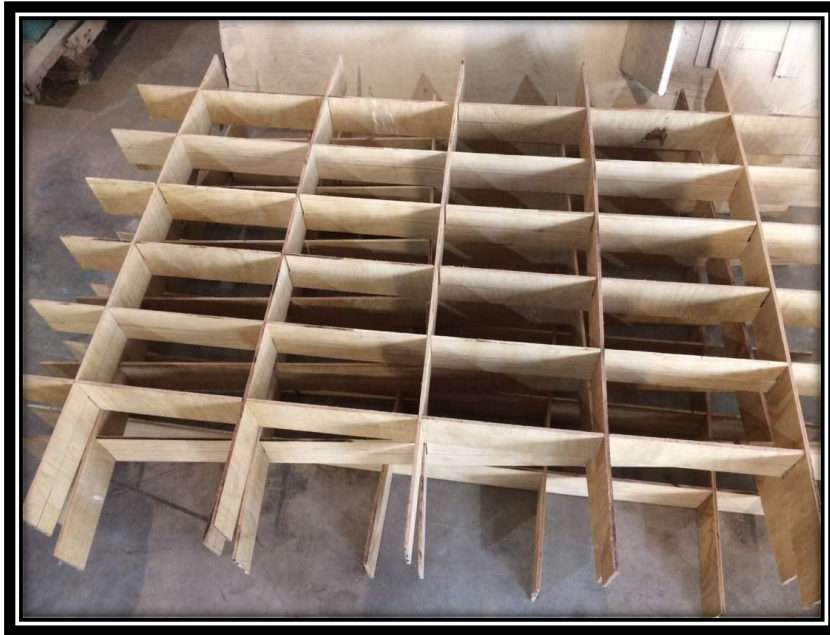
Figure 3.11 The formwork after the piece of plywood installed together
