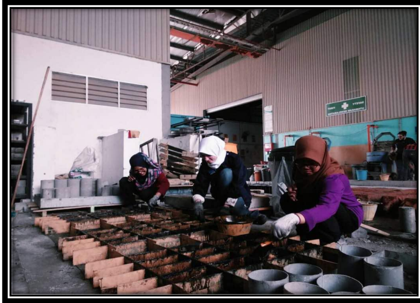
Figure 3.13 The formwork are painted using oil
