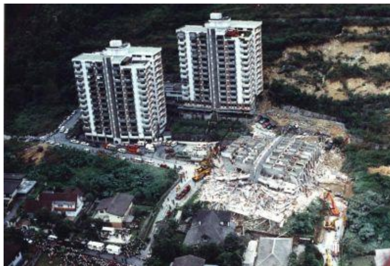
Figure 2.9 One of apartment at Highland tower was collapses due to slope failure
