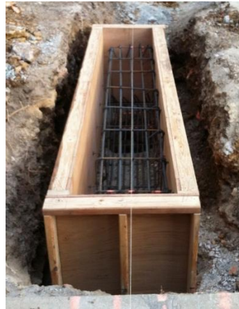
Figure 3.7: Beam formwork
