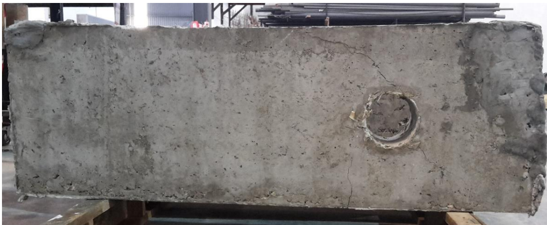
Figure 4.18: Cracking pattern for beam contain 1% of hybrid fibre
