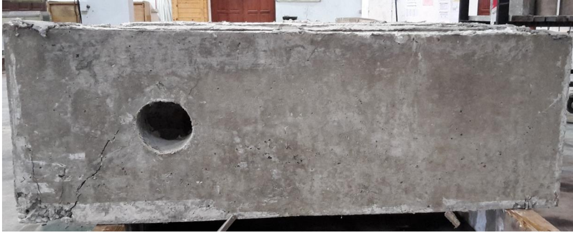
Figure 4.19: Cracking pattern for beam contain 2% of hybrid fibre
