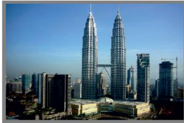
Figure 2.2: Petronas Twin Tower.
