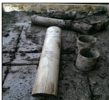
Figure 3. Installation of cement columns using PVC tube
