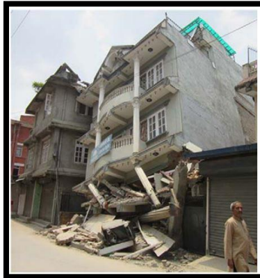
Figure 7. Low rise RC frame building due to the 2015 Nepal earthquake [13]
