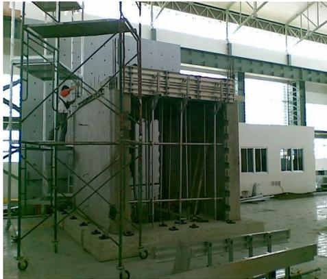
**Figure 1.** Cast-in-situ beams and slabs are used to joint two wall panels.
