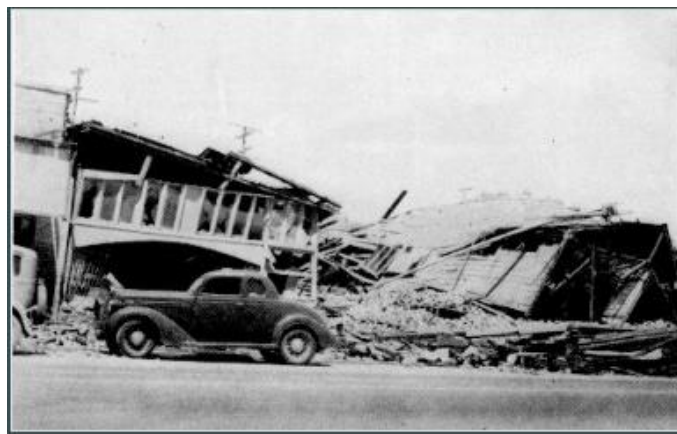
Figure 2.9 The collapse of these walls in the business district of Imperial caused the deaths of four people.
