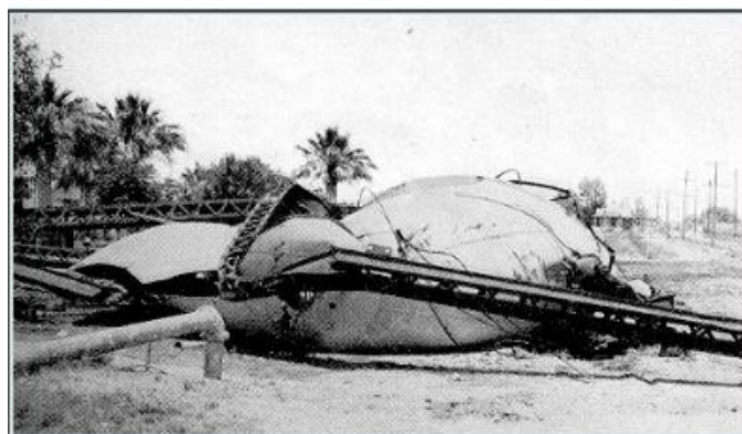
Figure 2.10 The collapse of the 100,000 gallon city water tank at Imperial.
