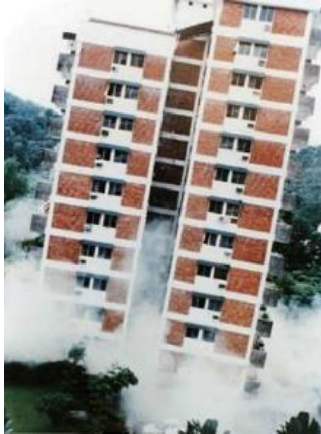
Figure 2.23 Highland Towers during collapse. Source: Jamie (1993).
