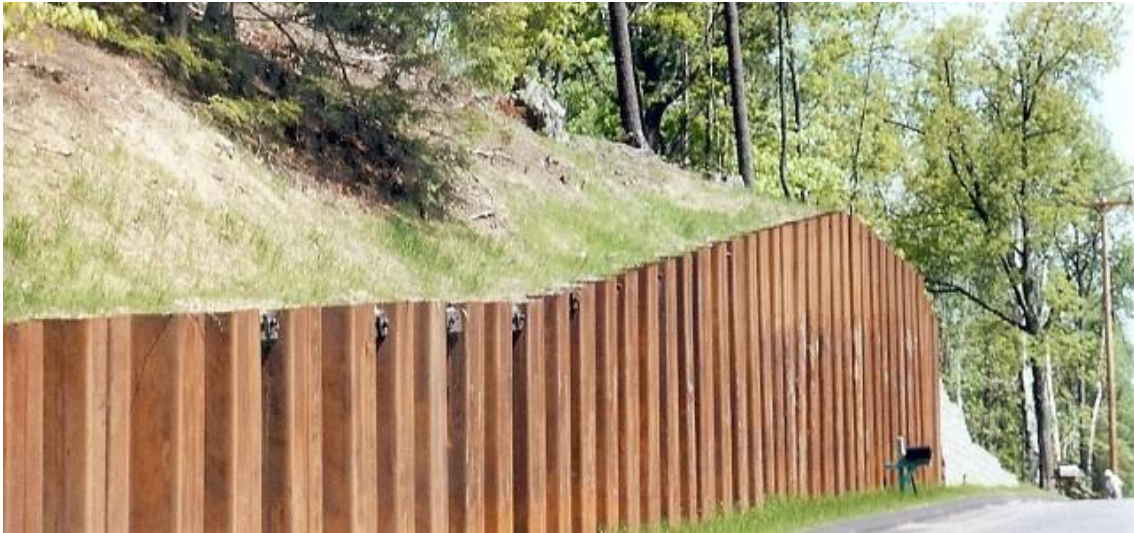
Figure 2.27 Sheet pile retaining wall.
