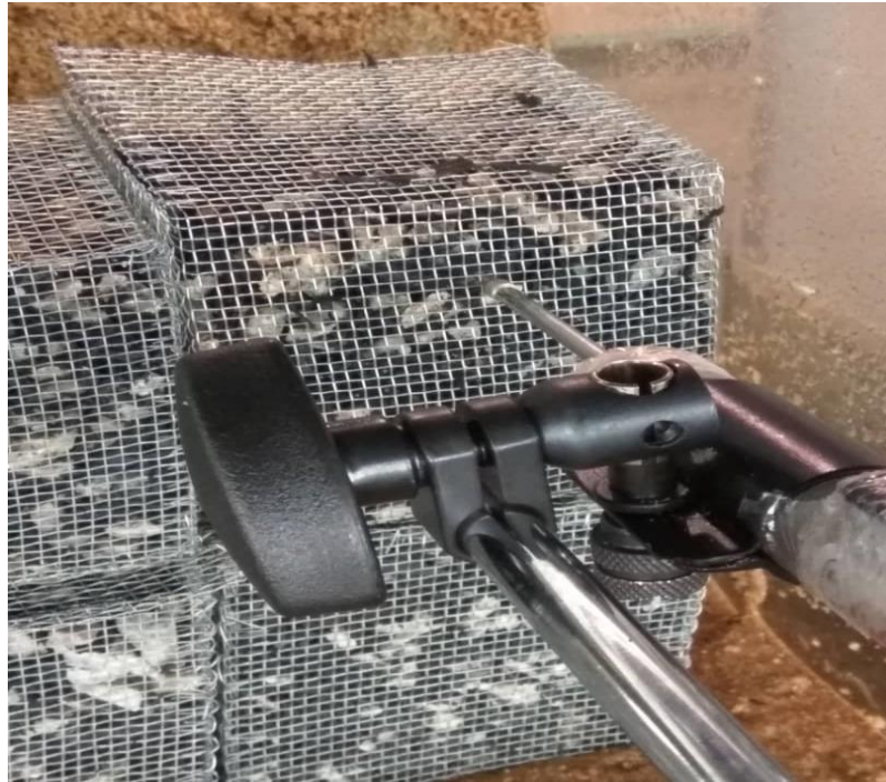
Figure 3.4 Digital transducer was used to measure the movement of gabion wall
