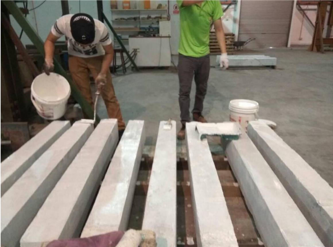
Figure 3.10 Painting of the Beams
