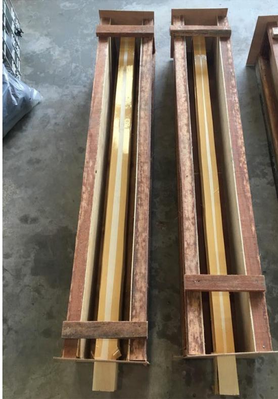
Figure 3.2 Preparation of Formwork
