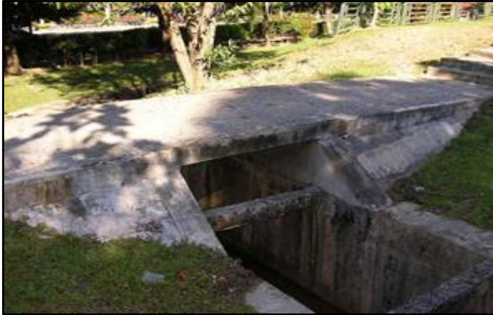
Figure 2.11 Foot-bridge structures made from OPS concrete.
