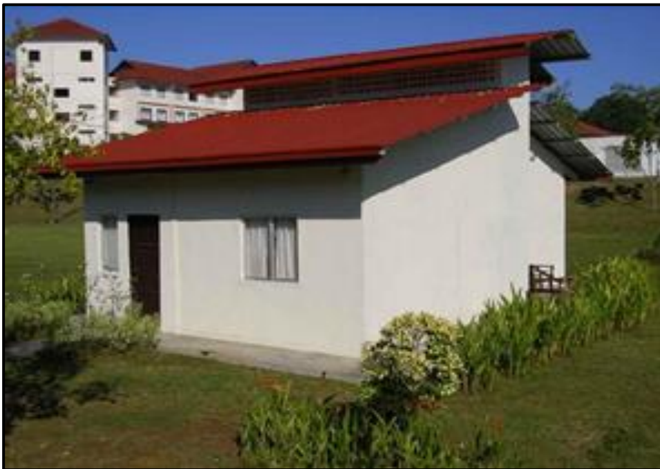
Figure 2.12 Low-cost house structures made from OPS concrete.
