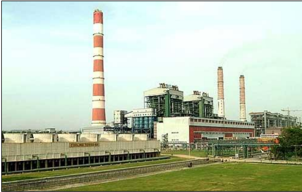
Figure 2.1 Vindhyachal Thermal Power Station, Madhya Pradesh
