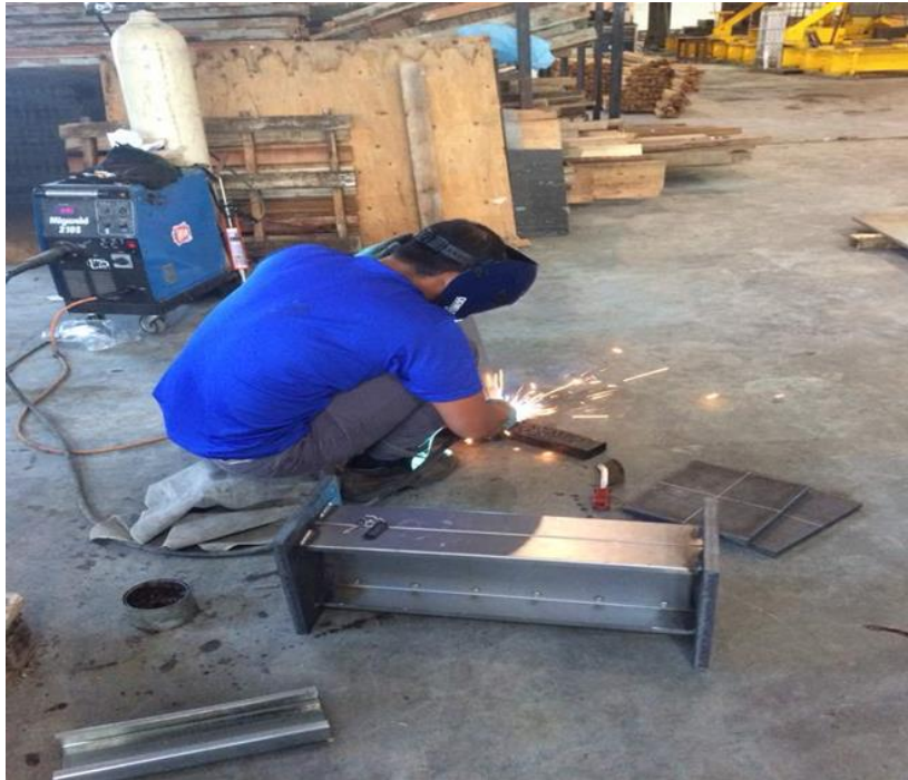
Figure 3.9 Process to welding the plate
