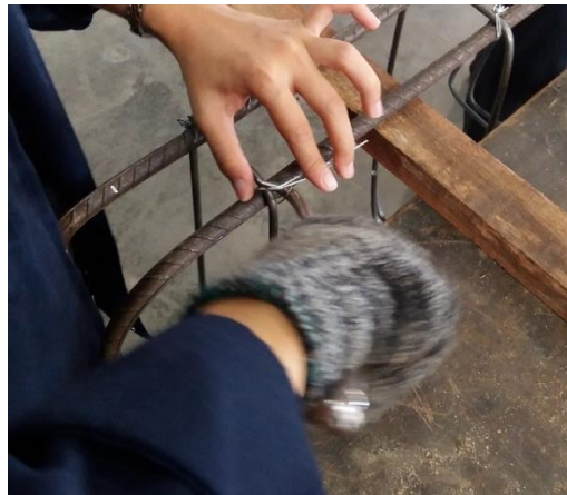
Reinforcement set up
