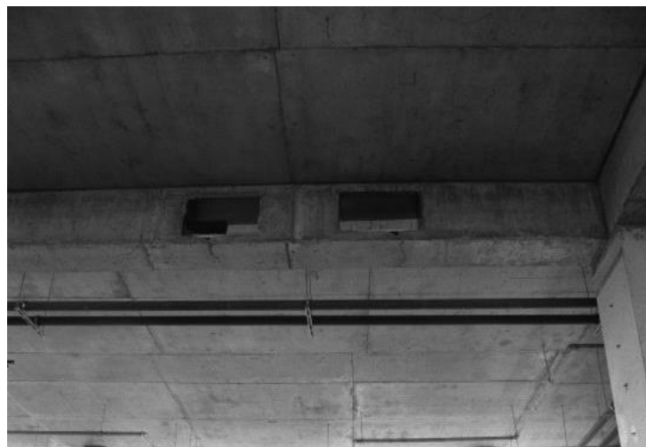
Figure 1.1 Multiple opening in a beam
