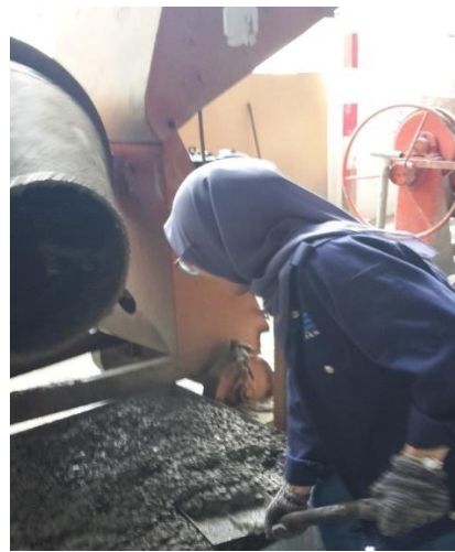
Mixing and casting
