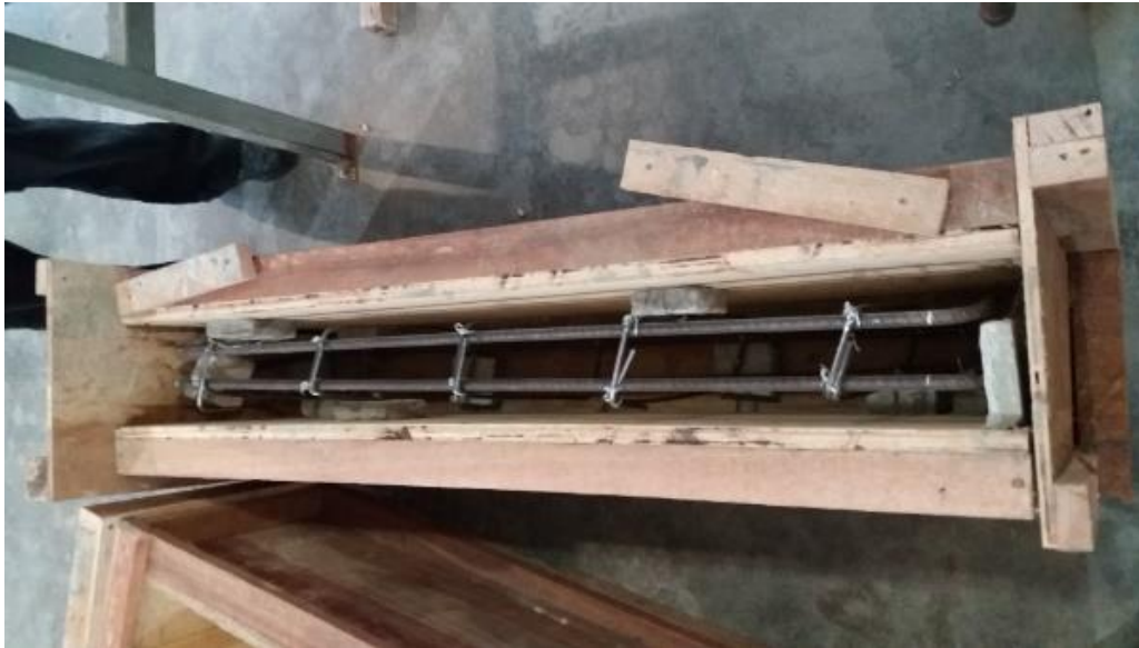
Figure 3.7 Beam formwork using plywood
