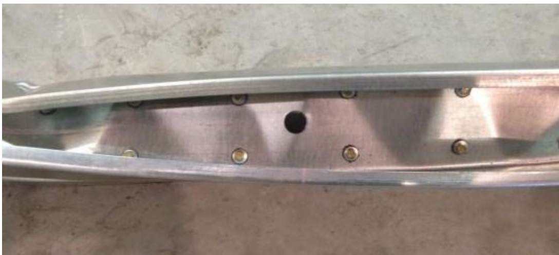
Figure 4.8 Local buckling at the middle of the beam after experiment (post – peak)
