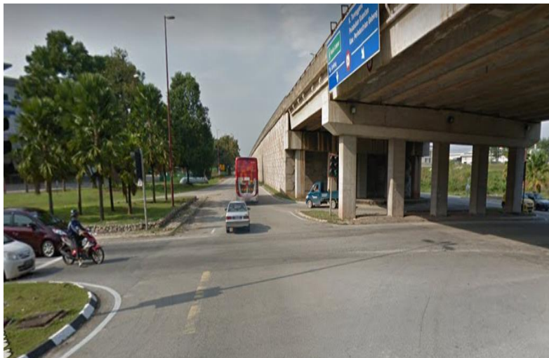
Figure 3.4 The signalize intersection of Wisma Belia
