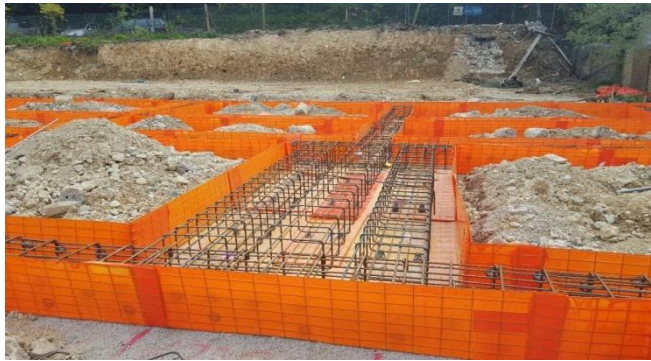
Figure 2.3 Permanent Formwork
