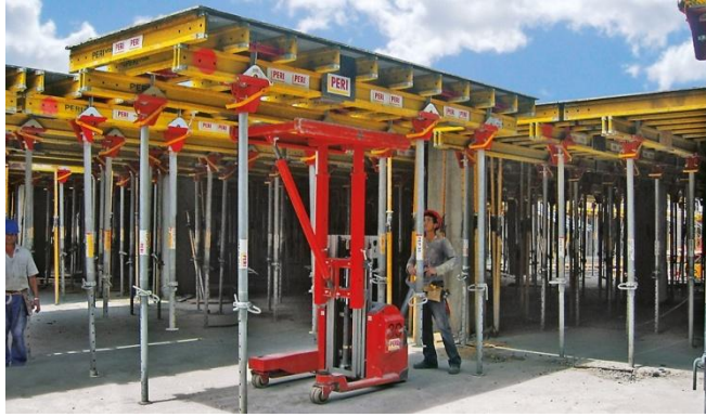
Figure 2.4 Table Formwork
