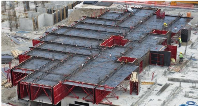
Figure 2.5 Tunnel Formwork
