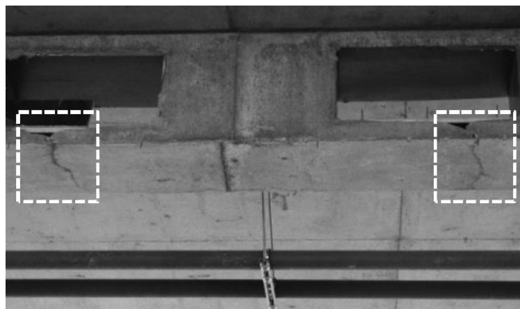
Figure 1.3 Failure at Opening of Beam Source: Zdanowicz & Wojdak (2013)
