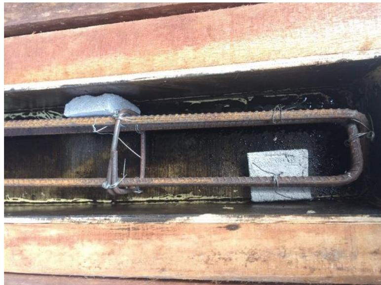
Figure 3.11 Spacer blocks tied with rebars.
