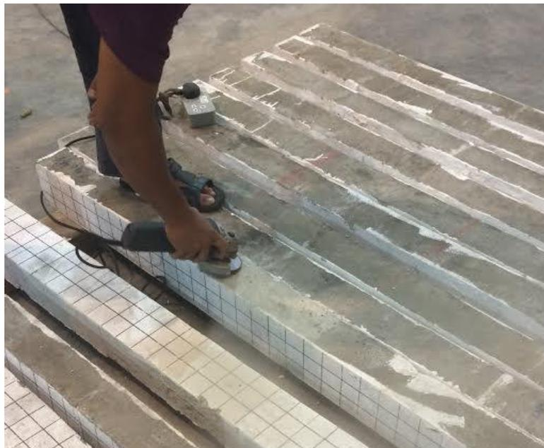
Figure 3.16 Roughening surface of RC beams.
