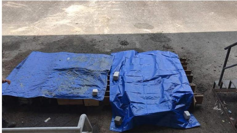
Figure 3.14 Cover the beam with canvas after pouring of concrete.
