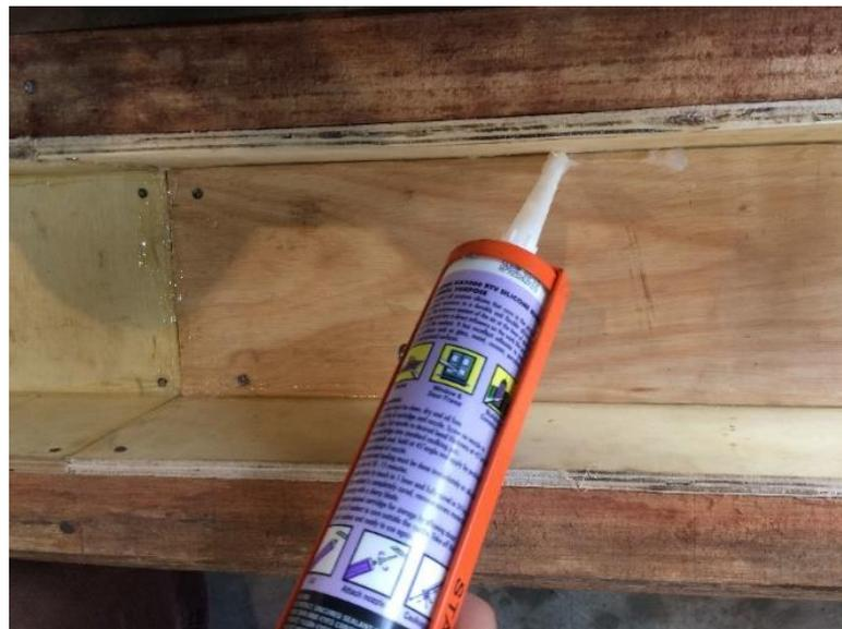
Figure 3.8 Sealing of formwork.
