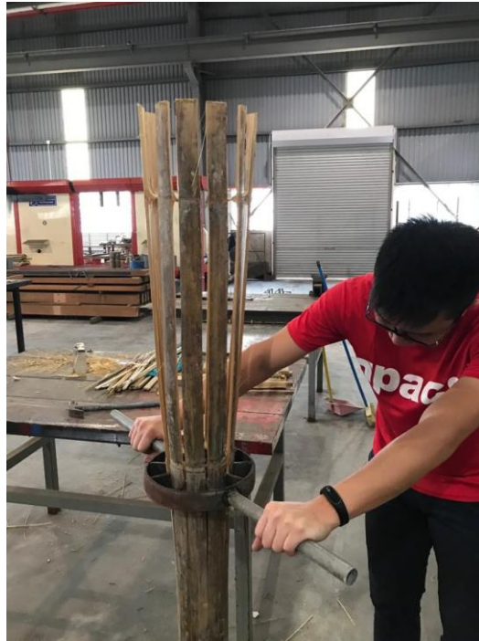
Figure 3.5: Splitting of bamboo culm
