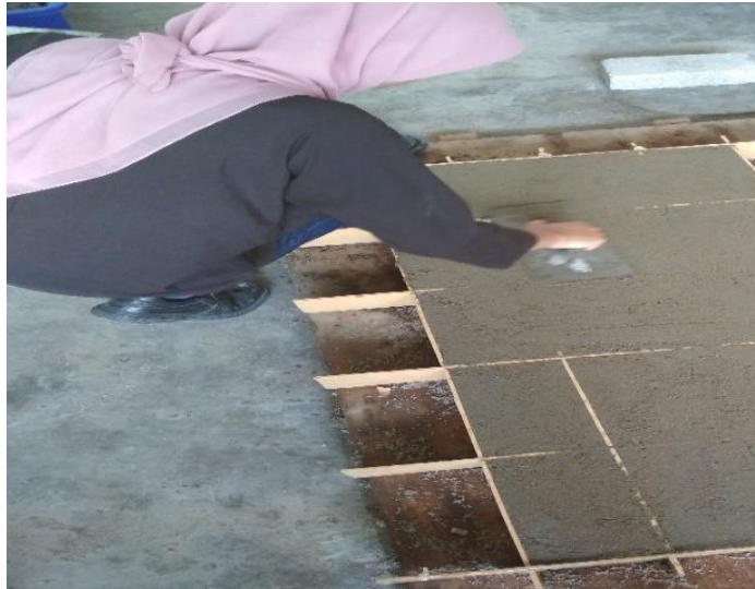
Figure 3.12 Brick casting already done
