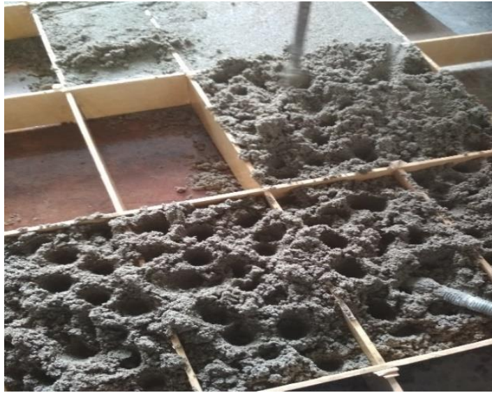
Figure 3.11 Process of placing brick mixture into formwork
