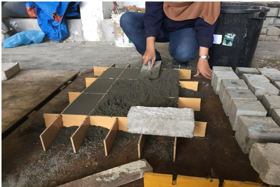
Figure 3.7 The mix was pour into the wood mould
