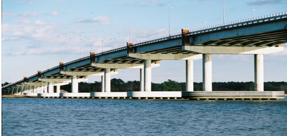
Figure 2.2: Bridge that built using lightweight aggregate concrete
