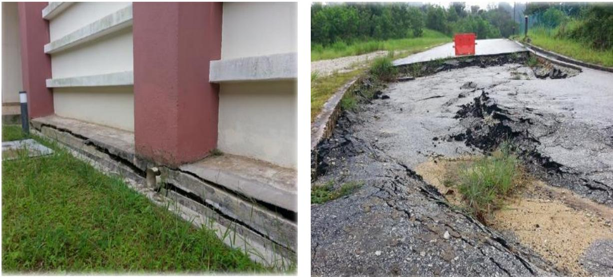
**Figure 1.** Existing Slope Location (Building & Road Damaged Signs)
