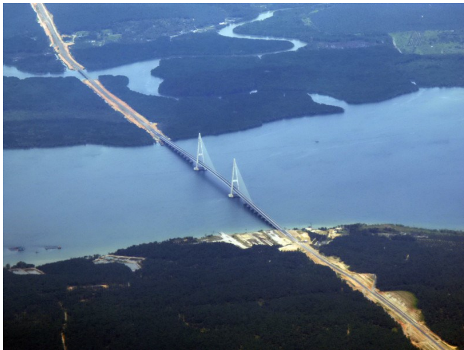
Figure 2.23 Johor river Bridge , Johor
