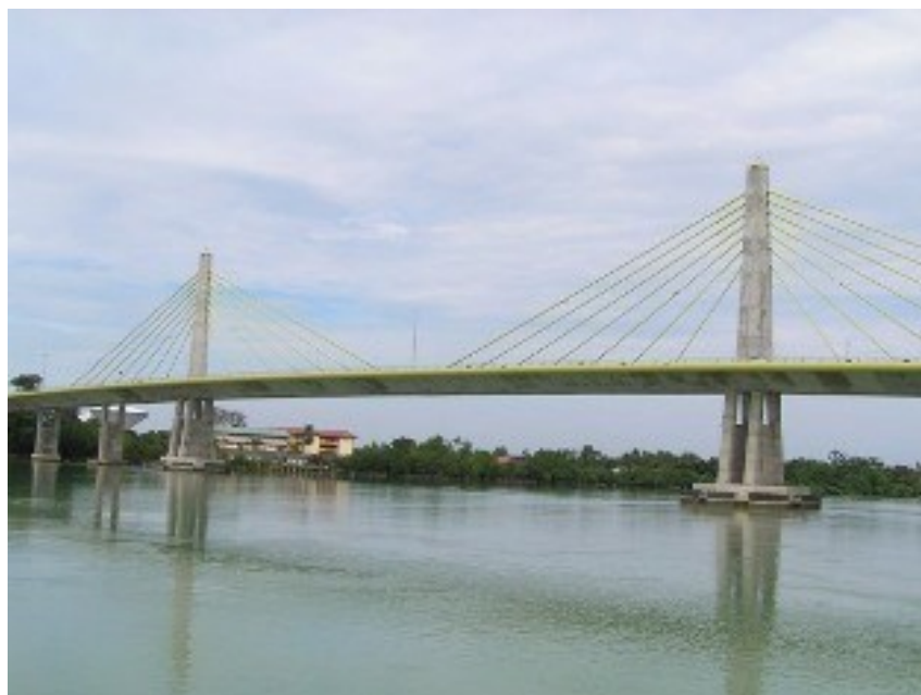
Figure 2.17 Muar Second Bridge, Johor
