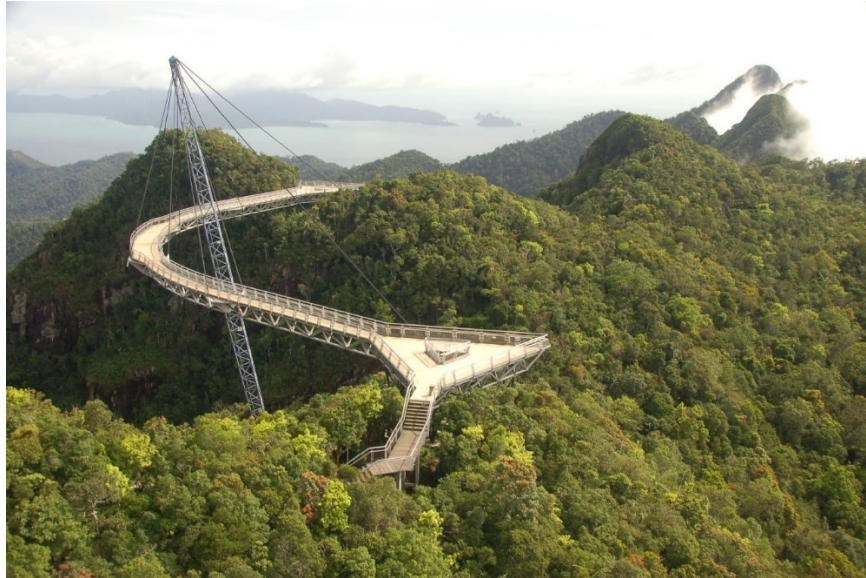
Figure 2.16 The Langkawi Sky Bridge , Kedah
