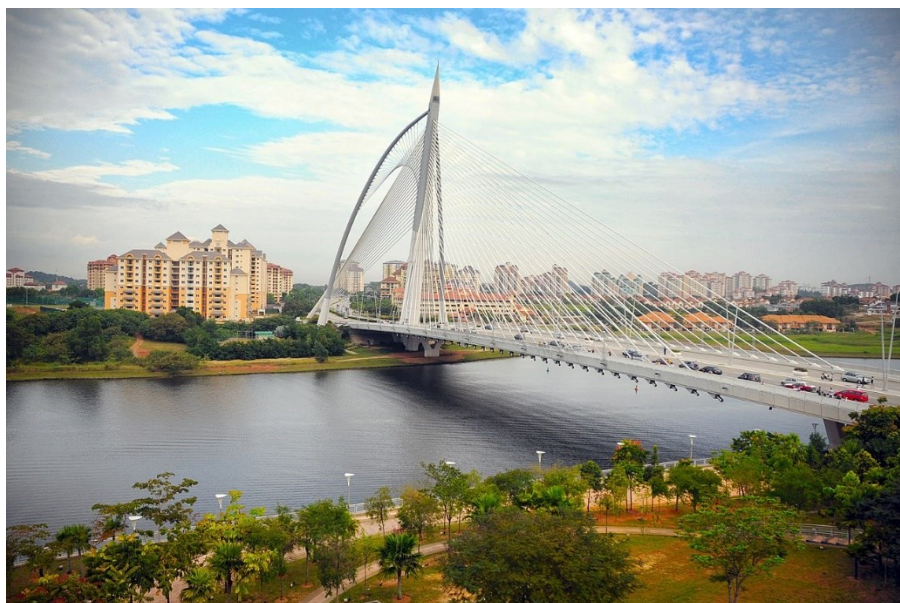
Figure 2.21 Seri Wawasan Bridge, Putrajaya
