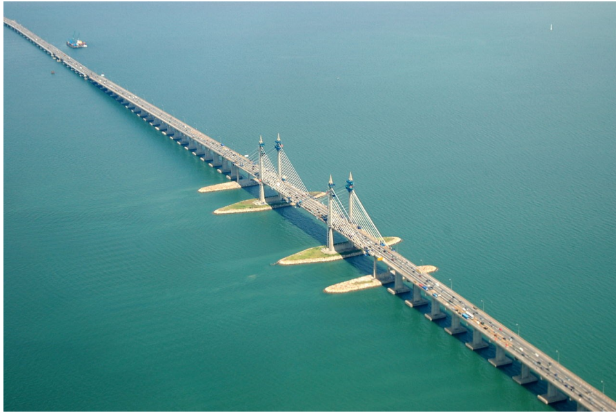
Figure 2.22 Sultan Abdul Halim Bridge, Penang
