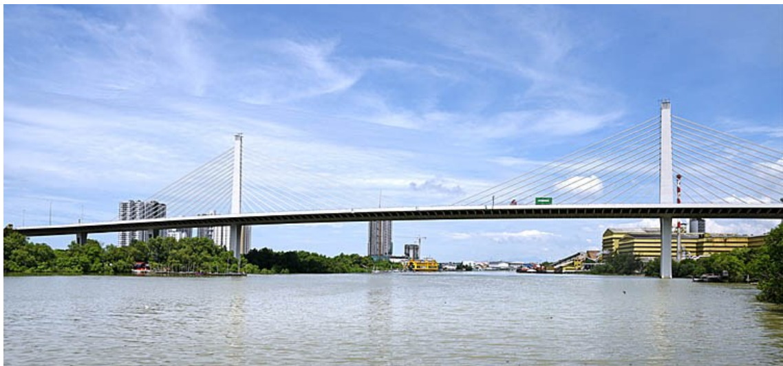
Figure 2.19 Prai River Bridge, Penang
