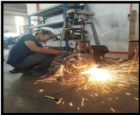
Cutting the Reinforcement Bar
