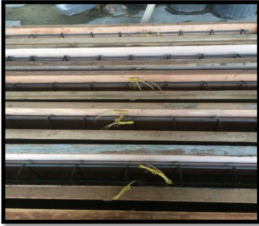
Strain Gauges Installation
