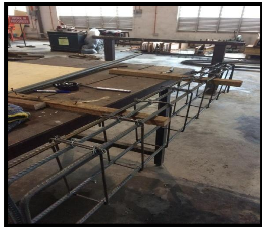
Installation of Reinforcement Bar
