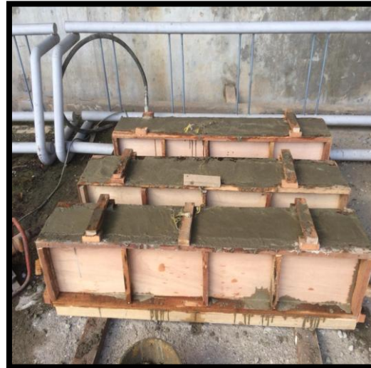
Concreting Work Done
