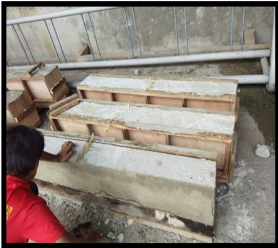
Formwork Removal
