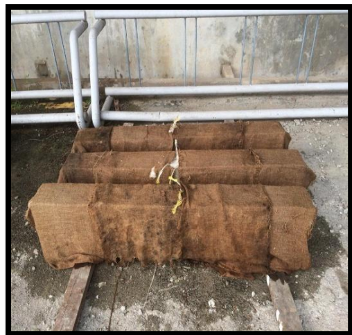
Curing by Using Wet Gunny
