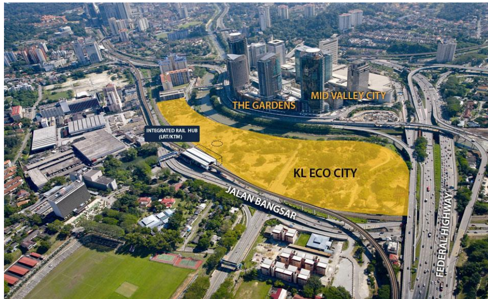
Figure 2.2 KL Eco City Aerial View
