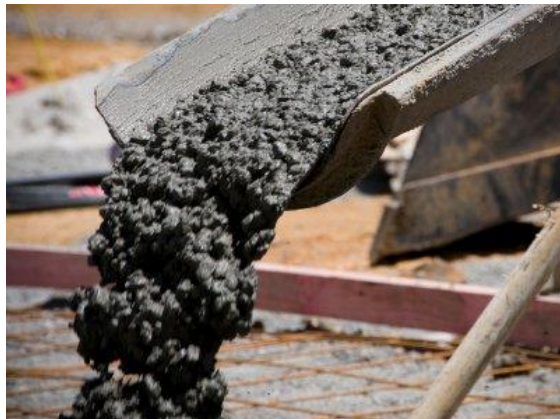
Figure 2.7 shows an example of Concrete mixing
