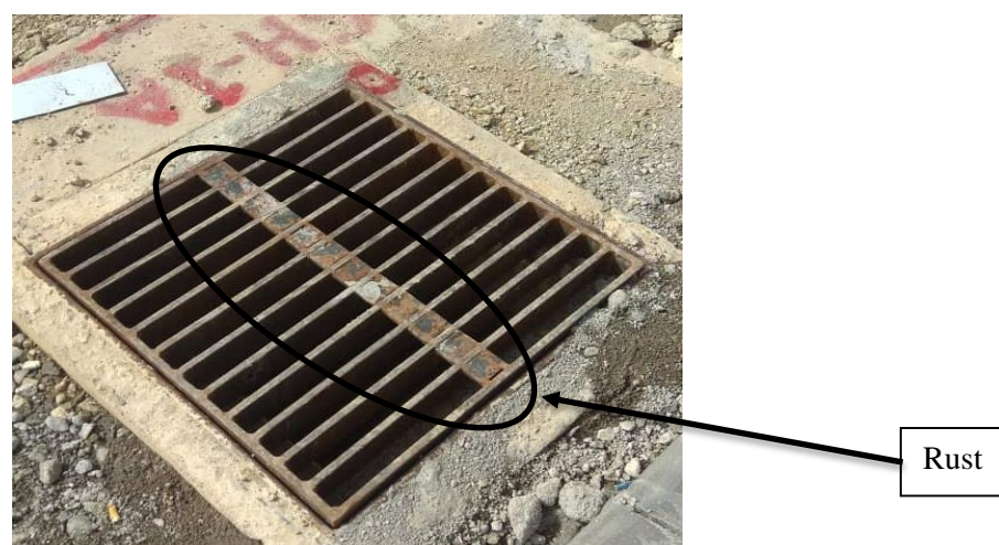
Figure 2.7 Rusty Manhole Cover at Timurbay Site, Kuantan Pahang (Fieldwork, 2018)
