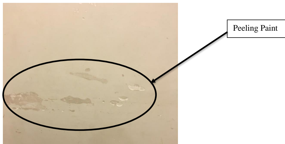
Figure 2.5 Peeling Paint Defect at East Coast Mall Kuantan, Pahang (Fieldwork, 2018)
