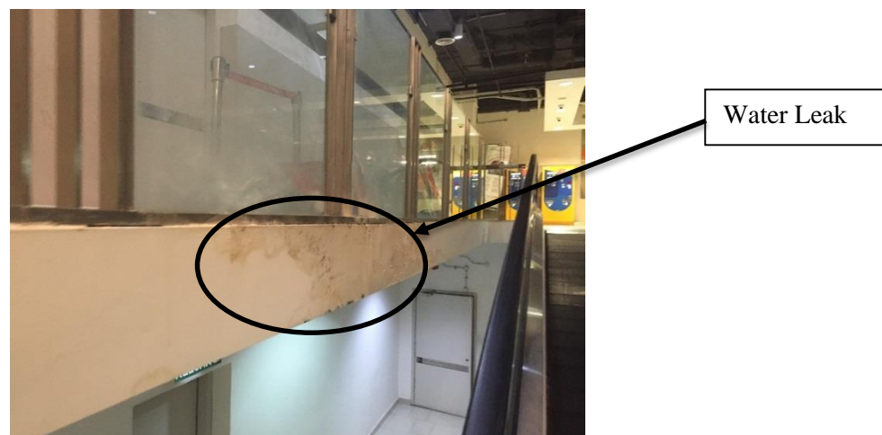
Figure 2.8 Water Leaking Defect in Paradigm Mall, Johor Bharu (Fieldwork, 2018)
