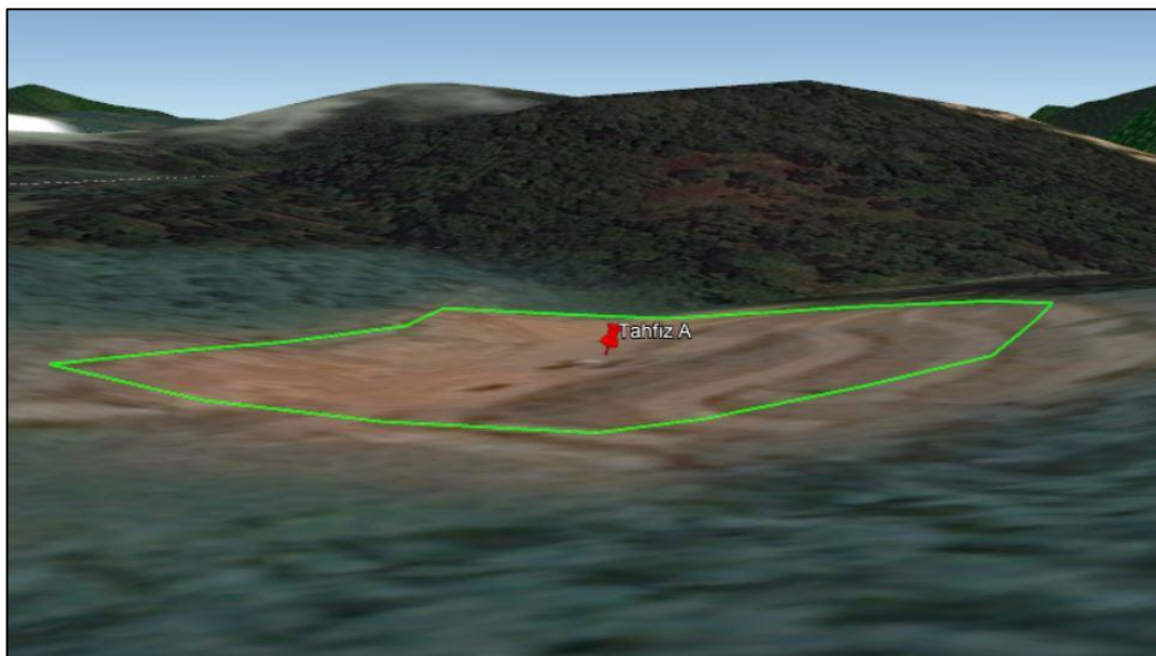
Figure 4.2 Position and view of slope at Tahfiz A
