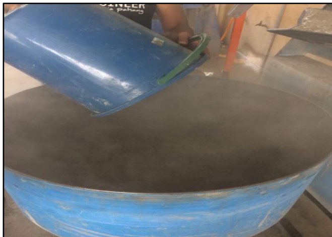
Figure 3.11 Pour materials into concrete mixer pan
