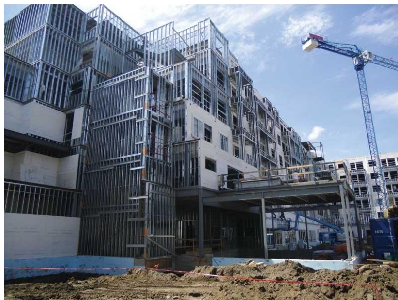
Figure 1.3 Cold-formed steel framing
