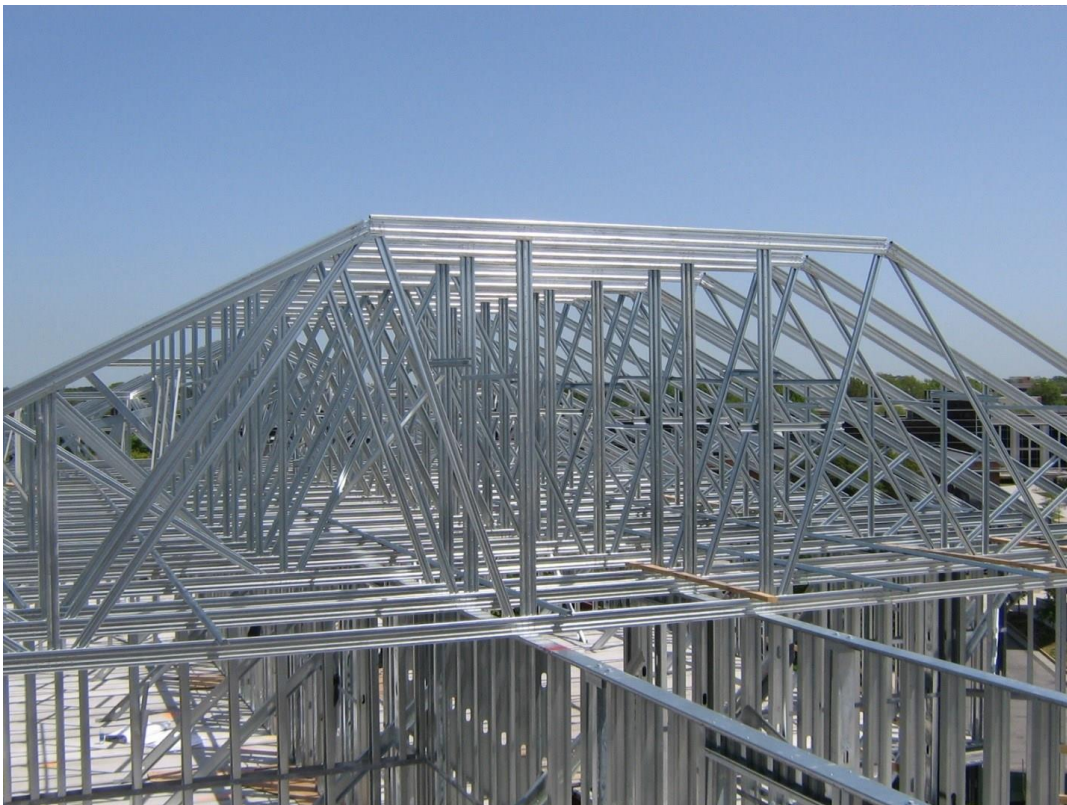
Figure 2.2 Cold-form steel roof trusses
