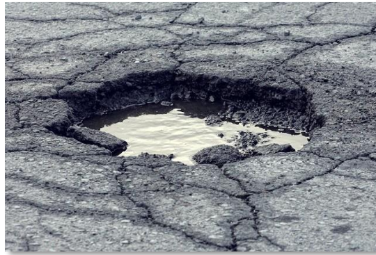
Figure 2.4 : Potholes
