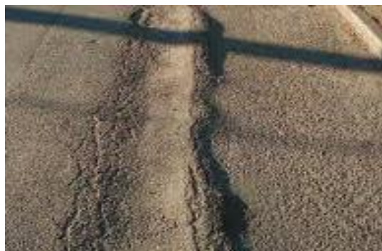
Figure 2.5 : Rutting
