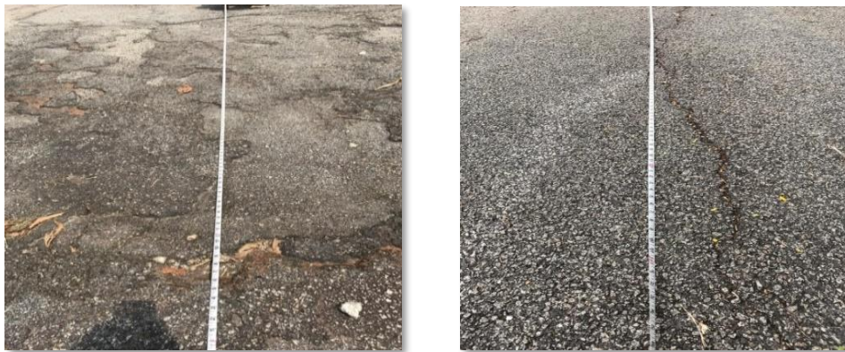
Figure 4.9 : Cracking
