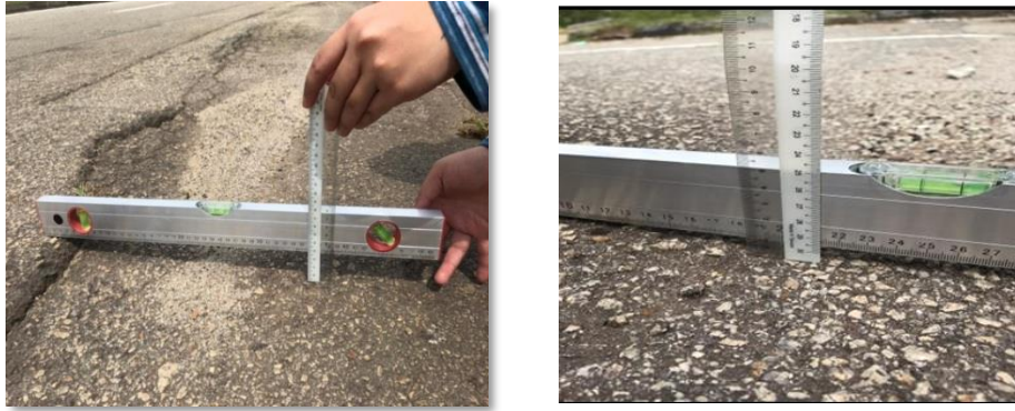
Figure 4.10 : Rutting
