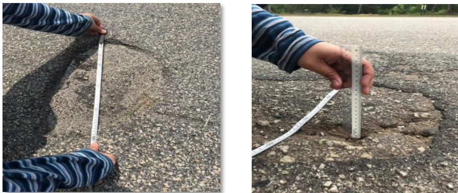
Figure 4.11 : Potholes
