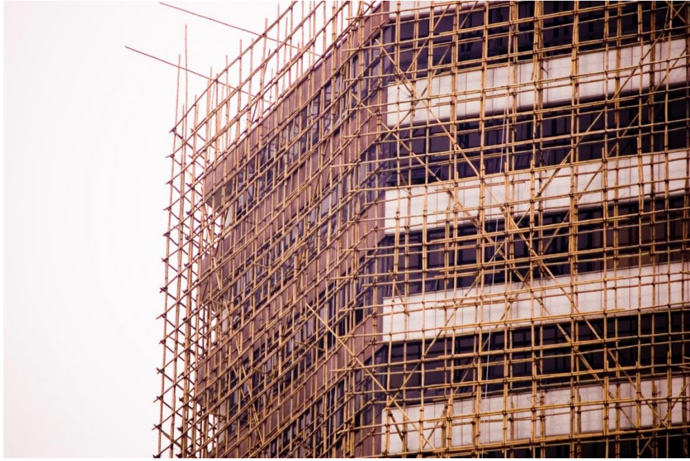
Figure 2.3 Bamboo scaffolding used to build Hong Kong Skyscrapers
