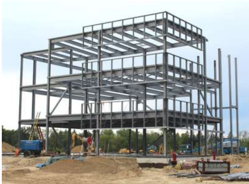
Figure 1.1 Steel frame structure
