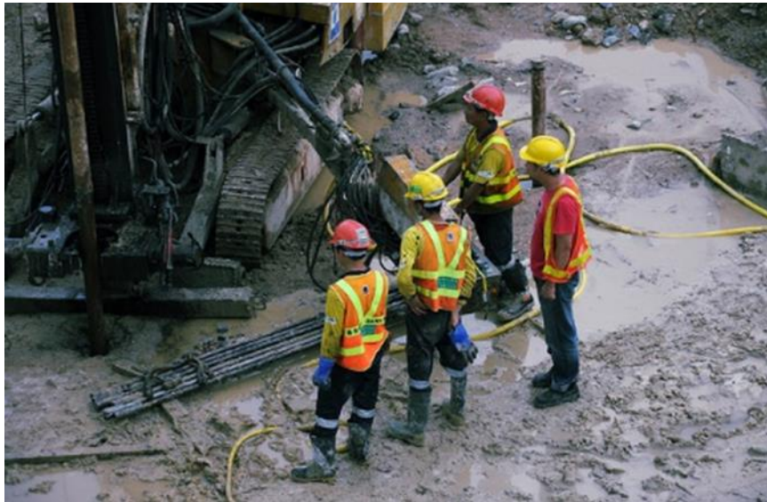
Figure 2-4: Raining Season May Affect the Work Progress
