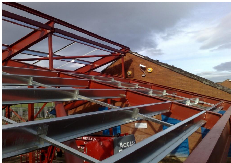
Figure 2.1 C-section of CFS for purlins at the roof system (Source: https://mtc-china.com/steel-purlins/ )
