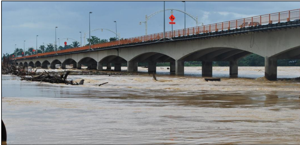
Figure 1.1 Sultan Yahya Petra Bridge, Kelantan
