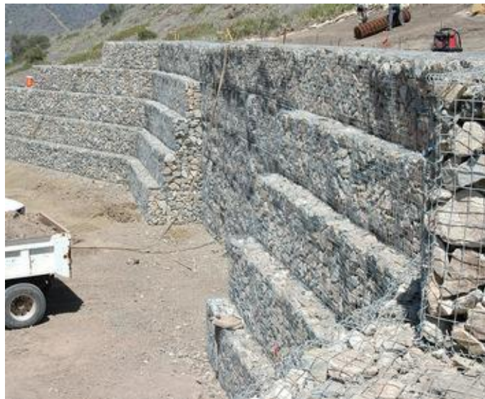
Figure 2.13 Application of gabion wall at cut slope.
