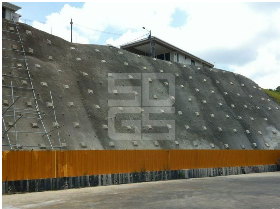
Figure 2.9 Application of soil nailing in the field.
