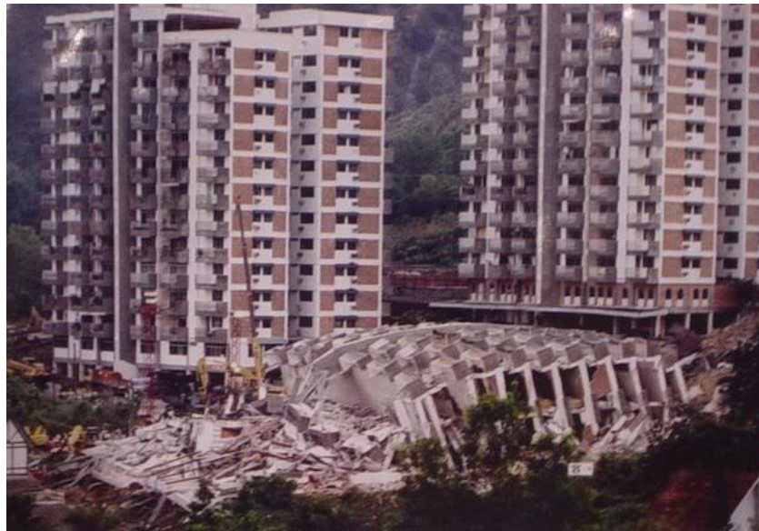
Figure 2.5 Highland tower collapse.
