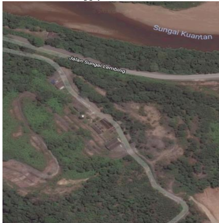
Figure 6.3 Location of Sg. Lembing WTP
