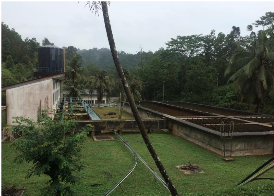
Figure 4.1 Sg. Lembing Water treatment Plant
