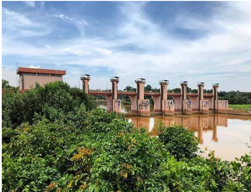
Figure 4.16 Semambu Water Treatment Plant
