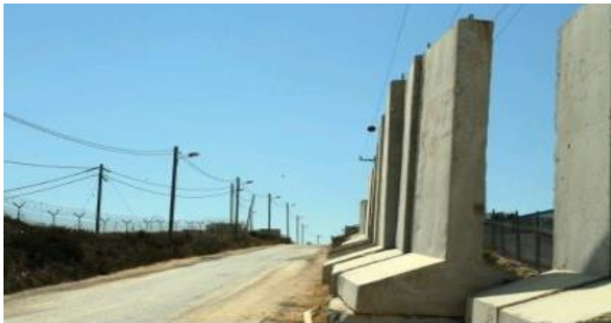
Figure 1.1 Typical RC wall
