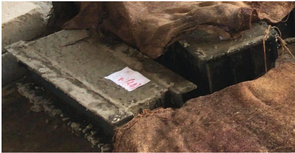
Figure 3. 7 : Concrete Beam Mould
