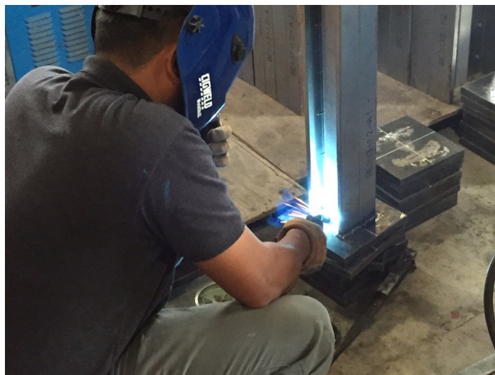
Figure 3. 4: Welding work of specimens
