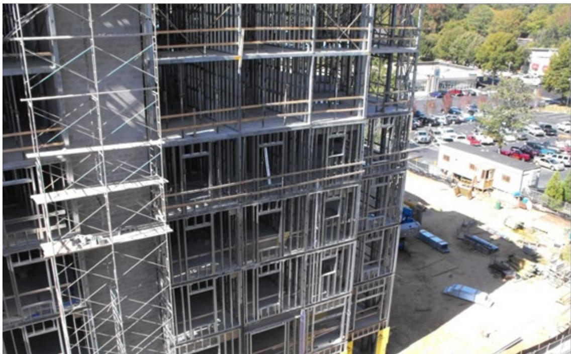
Figure 1. 2: One of the usage of cold-formed steel
